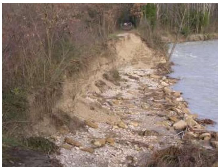
PHOTO 16 : EROSION DE LA DIGUE D'ENTONNEMENT D'ALLEX
