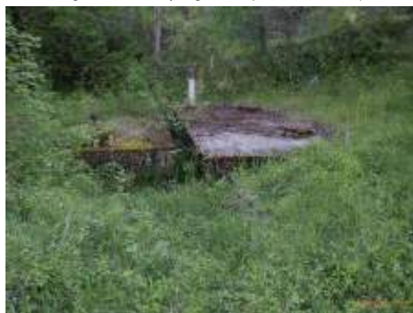
Figure 132 : captage AEP (26CCVD0041)
